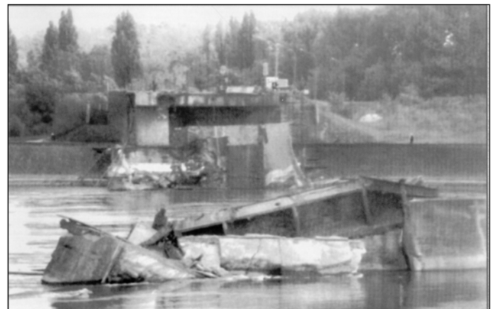
Fig. 3. The Zezelj bridge (km 1254.17) prior to destruction on April 26 th 1999 (on the left), and at the end of 2001 (on the right); its prestressed concrete arch structure had 231 m and 180 m spans; in spite of numerous echo soundings, the exact position of arches lying on the riverbed is still unknown, but it is estimated that a 7 m high underwater sill has been formed along the entire cross section, radically affecting the flow pattern.
