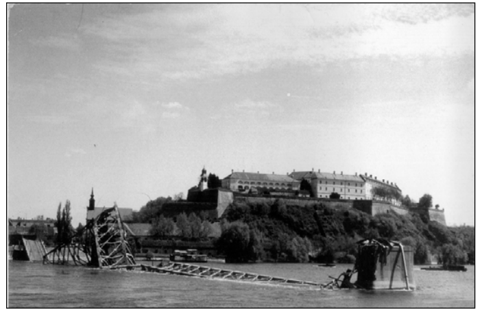
Fig. 2. The Petrovaradin bridge (km 1255) before destruction (on the left), and after destruction (on the right); its structure was K-type girder truss, with the central span of 130 m, and two minor spans 51 m.
