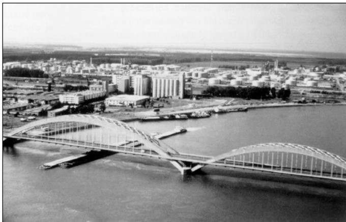
Fig. 3. The Zezelj bridge (km 1254.17) prior to destruction on April 26 th 1999 (on the left), and at the end of 2001 (on the right); its prestressed concrete arch structure had 231 m and 180 m spans; in spite of numerous echo soundings, the exact position of arches lying on the riverbed is still unknown, but it is estimated that a 7 m high underwater sill has been formed along the entire cross section, radically affecting the flow pattern.
