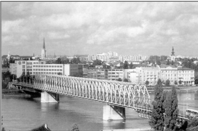
Fig. 2. The Petrovaradin bridge (km 1255) before destruction (on the left), and after destruction (on the right); its structure was K-type girder truss, with the central span of 130 m, and two minor spans 51 m.
