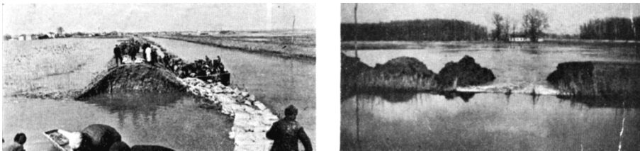
Figure 1.4: Reparation of a Danubean levee near city of Novi Sad, and a breach formed in the course of levee failure in April, 1940. [79]
